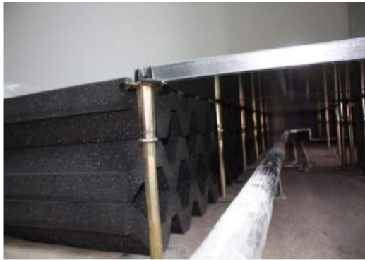
NAT Vent Attenuator Located under the raised floor used to control noise ingress
