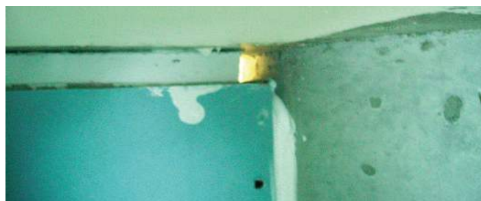
Gaps principally at the head and facade of partition interface. A major cause of on site shortfalls in sound insulation levels.
