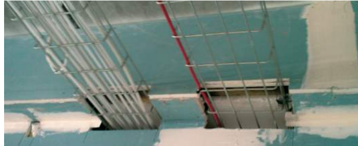
Cable tray passing through separating walls. This is impossible to acoustically seal.
