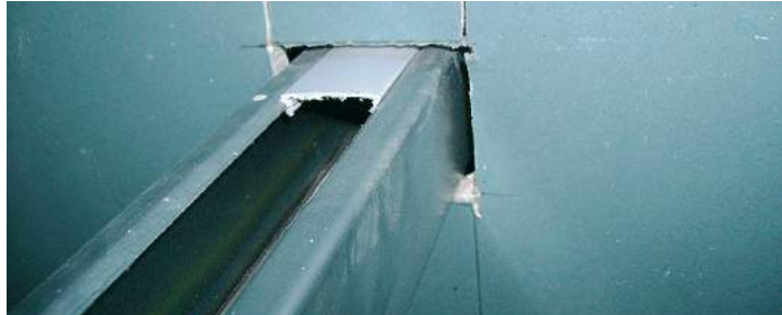
Electrical trunking not packed with sand bags, large gaps around the penetration point, no patressing
