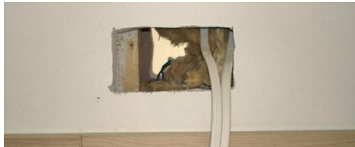
Back to back electrical sockets breaching the performance of the separating wall.
