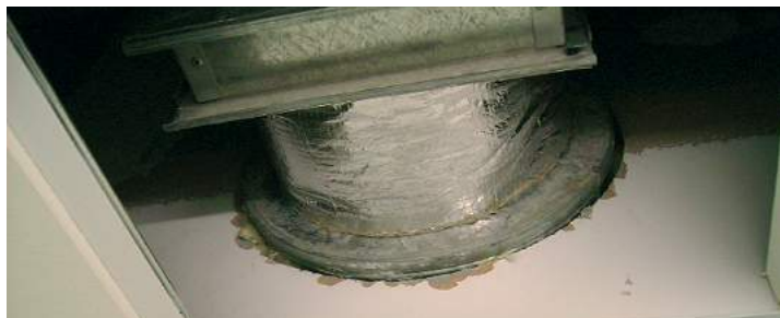
No patressing around cross talk attenuator, the cross talk should also straddle the partition, rather than installed on one side only.
