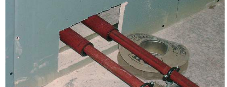
Pipe work hidden by raised floor, no patressing or sealing of any sort. Fails to meet acoustic requirements.
