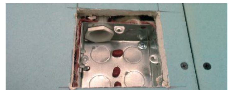
Acoustic putty poorly installed, still a large gap around the electrical socket.
