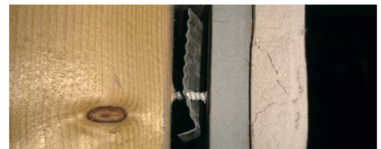
Incorrect screw size breaching the flexibility of the resilient bar and hence compromising the performance of this partition.
