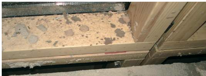
Junction between mullion and floor slab. The sealing between different constructions needs to be considered carefully to avoid large or awkward gaps which can be difficult to make good
